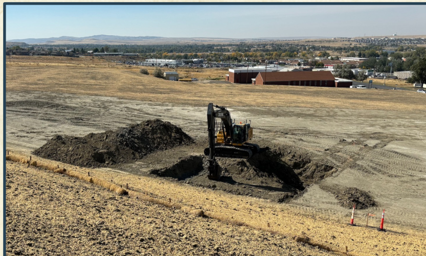
EXCAVATION OF FOUNDATION
